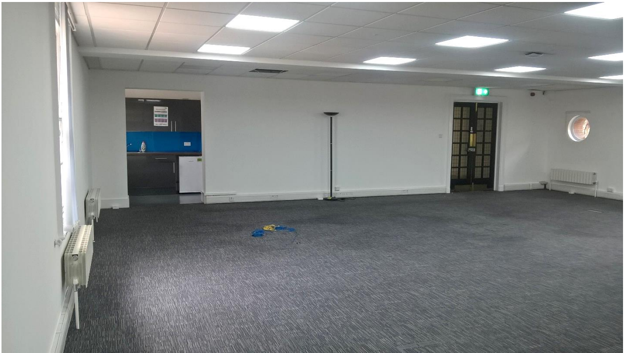
3 RD FLOOR B/C
