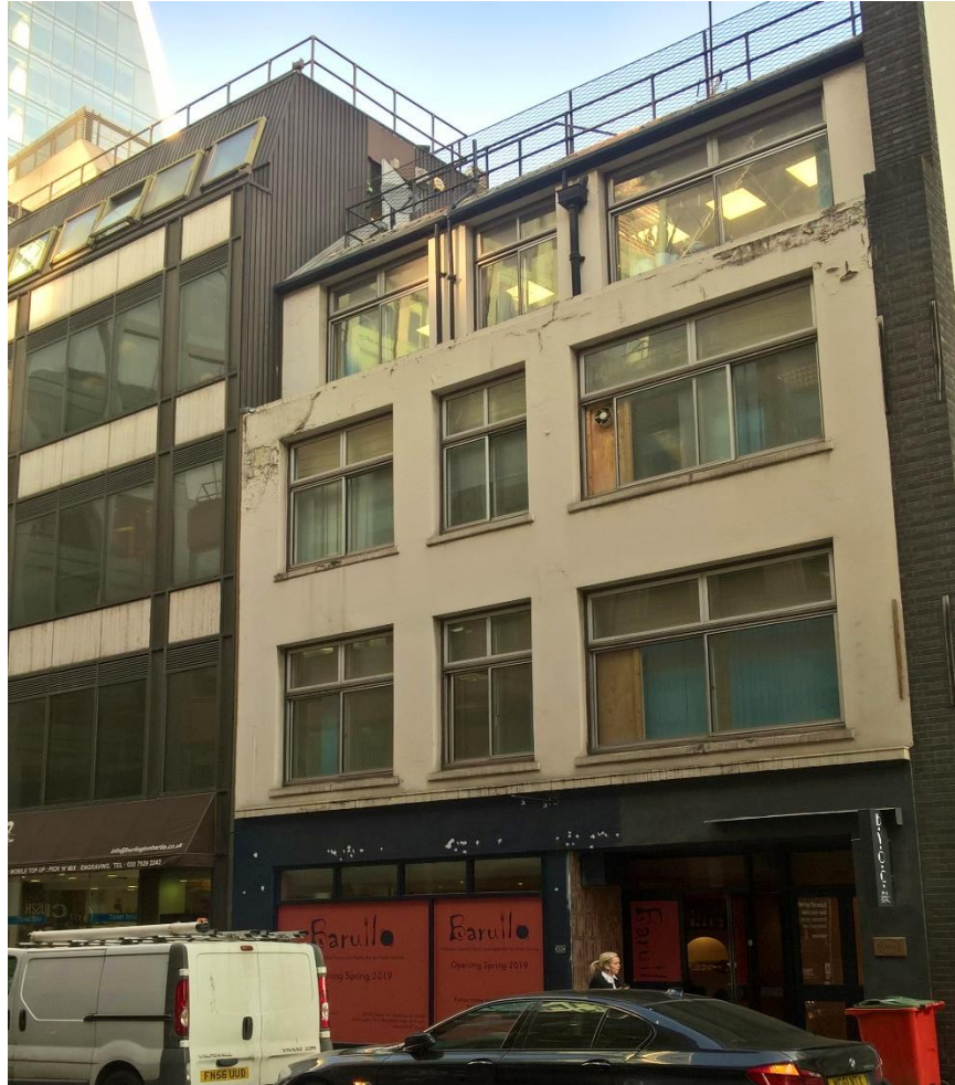
FRONTAGE TO BEVIS MARKS
